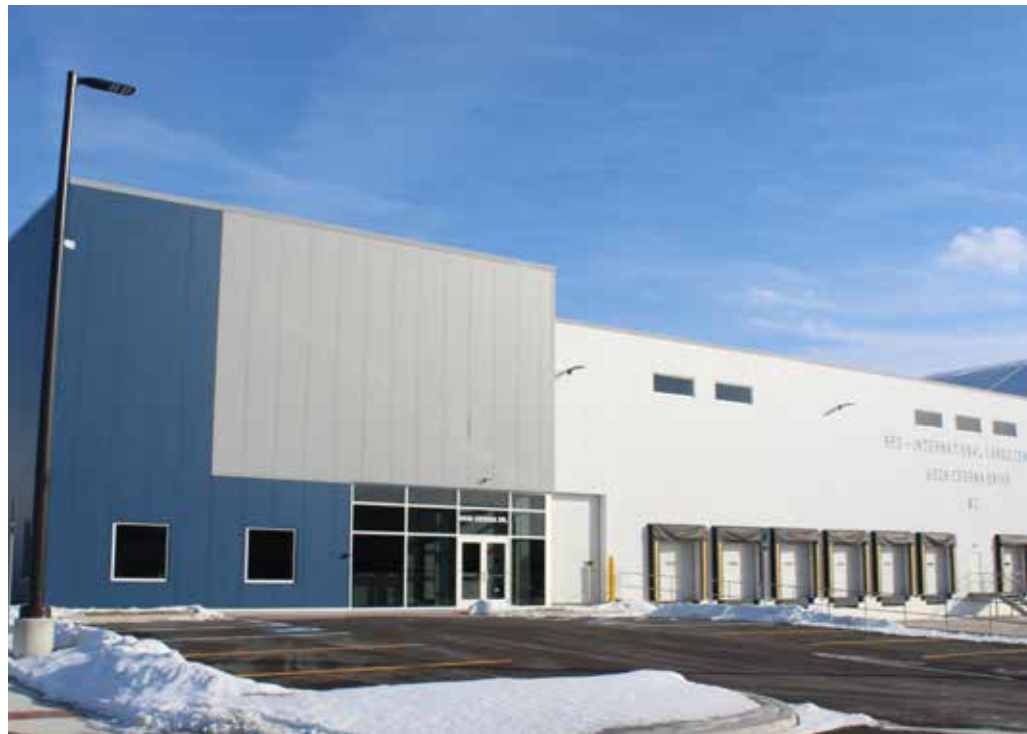
Last summer, Menzies took over RFD’s newest cargo building
