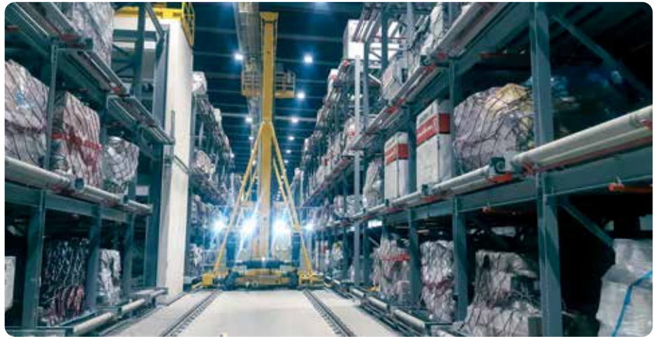
Turkish Cargo’s new IST facility includes automated high-bay warehouses with 17,000 storage locations, 30 stacking cranes, 15 lifts and an integrated warehouse management system
